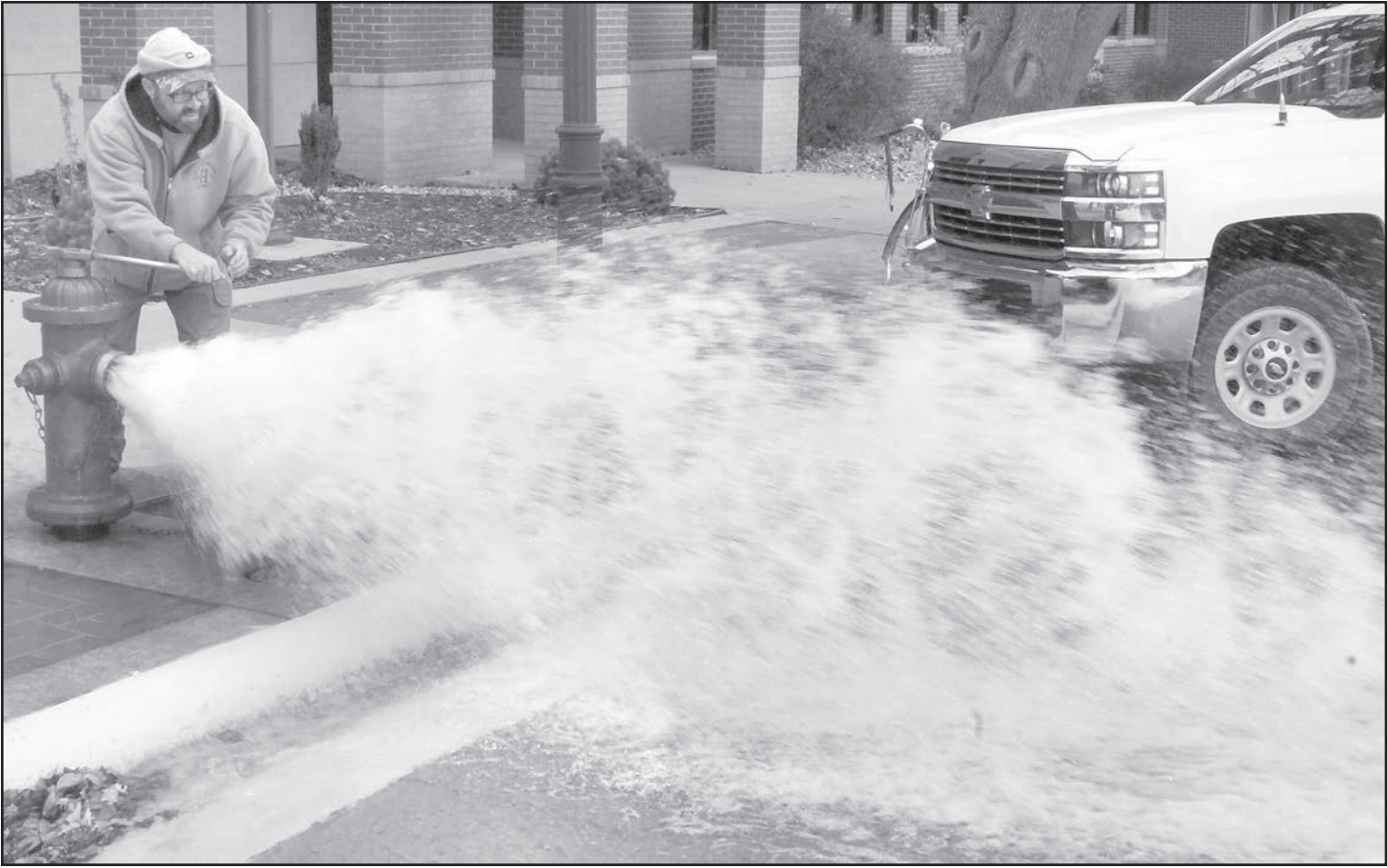
Holton city employee P.J. Oldehoeft turned on the fire hydrant in front of GNBank on Thursday to flush out the water lines in the vicinity of Hotel Josephine, just down the block from the bank. Oldehoeft said a “flow test” for the historic hotel was requested for fire protection purposes, and the test knocked some rust loose in the water lines, prompting the city to flush lines in the area.
