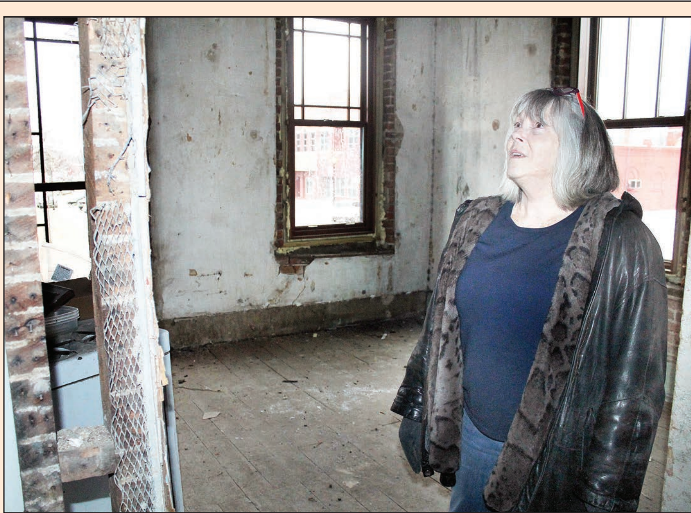
Colette Carson spent part of Friday overlooking improvements that have been made — and pondering those that have yet to be made — in the second-story space in the former Bernard Grocery building on the north-west corner of Holton's Town Square, where LaborMax Staffing now occupies the ground floor. Carson is also overseeing second-floor improvements in the adjacent Edward F. Jones building that houses the Fifth Street Sandwich Shoppe. Photo by Brian Sanders
