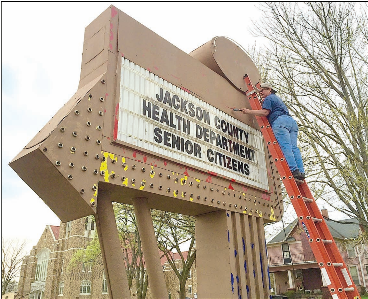
The big sign in Holton at 312 Pennsylvania Ave., the location of the Jackson County Health Department and Senior Citizens Center, is being repainted. Jill Bleier of Holton, shown above on the ladder, was scraping off loose, old paint from the sign on a recent day. Bleier said, from the top of the ladder, that the sign was a little higher off the ground than she originally thought it was when she bid on the work. “I’m the lucky one who got the bid,” she said. The sign, in its earlier days, advertised specials for Craig’s IGA and Mahon’s Shurfine grocery stores that were located there.
