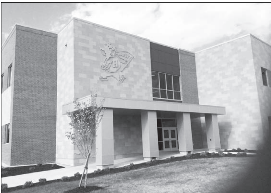
The top photo, taken inside the new Holton Elementary School, spotlights the school's multi-level media center, including its "Jim Lane Fort" and a huge mural on the center's east wall. The photo above shows the new school's west entrance, along with a Wildcat mural that appears on the school building. These and other notable features of the new school will be on display at the upcoming open house, scheduled for 3 p.m. Sunday, Oct. 23.
